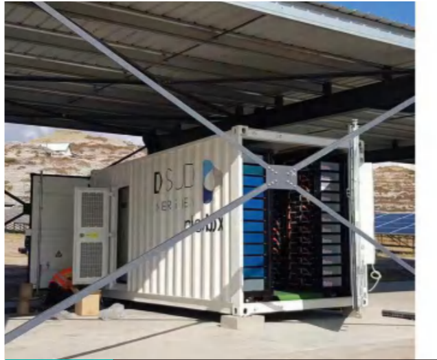
MADAGASCAR 1.5MWH/500KW Micro-grid Self-consumption ESS PV+DG+BESS
